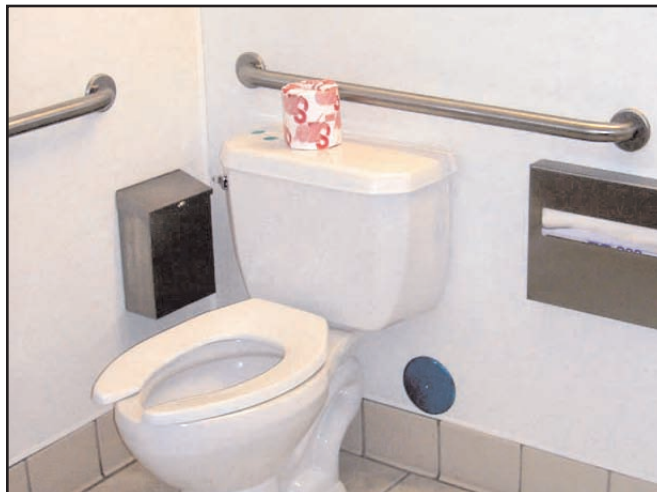
Grab bars behind and beside the toilet
