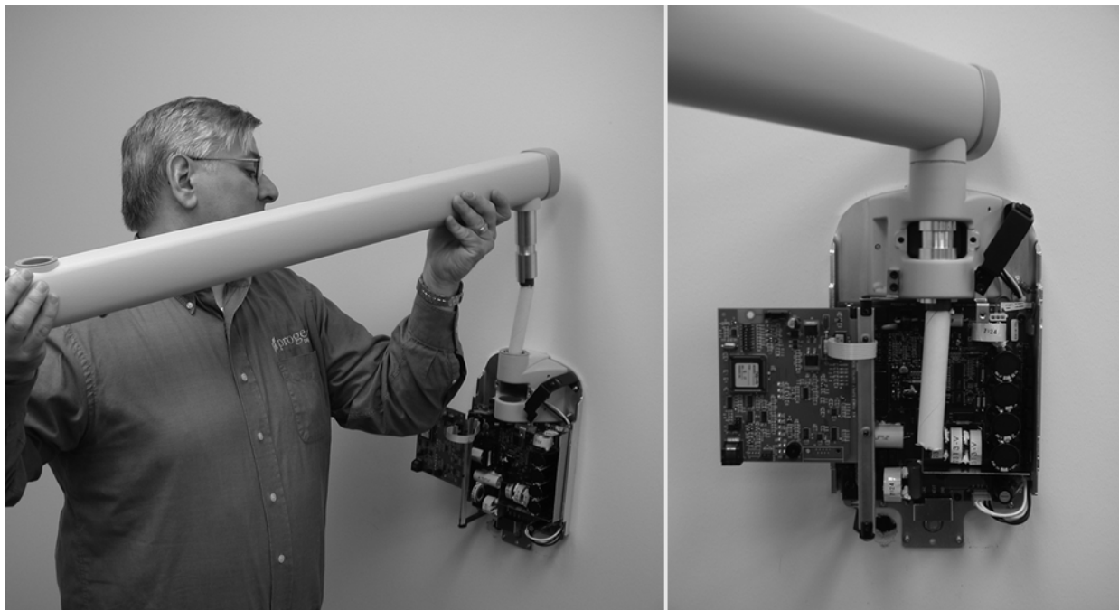
Figure 18 Installing the Horizontal Arm
