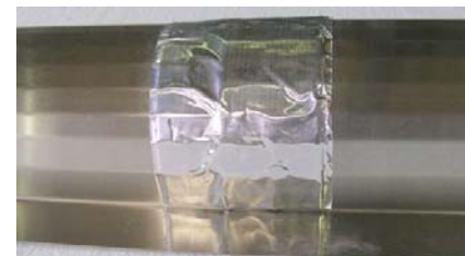
Drain Patch Fully Installed Figure 7D
