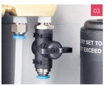
03 Water recycler bypass valve provides extra protection against water mineral deposits.
