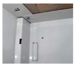
Mechanical fasteners (screws, pop rivets) and Tog-L-Loc<sup>®</sup> sheet metal joining system
