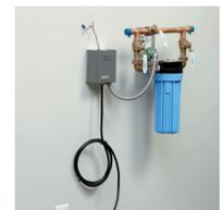
Water filter bypass separator
